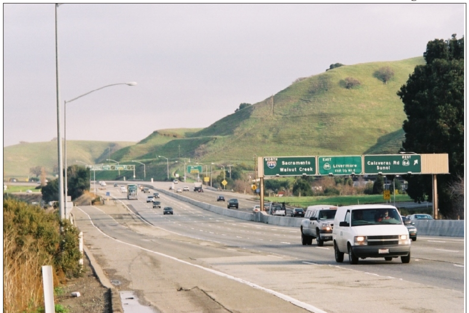
I-680 at SR 84 where the HOT lane will start
